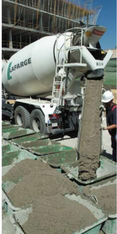
Stabilized MorPlast is a high quality plaster batched in Lafarge's concrete plant, delivered to site ready to use. No addition of water or other raw materials is required on site.
